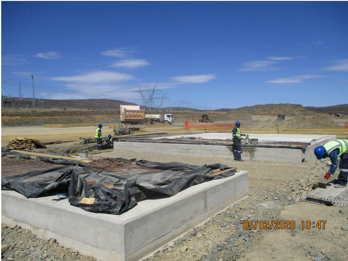
Photo: Preparation of shuttering at the transformer plinth.
