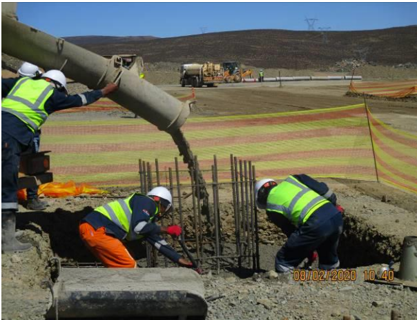
Photo: Casting concrete on foundation bases.
