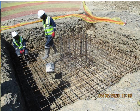
Photo: Steel fixing at the foundations.
