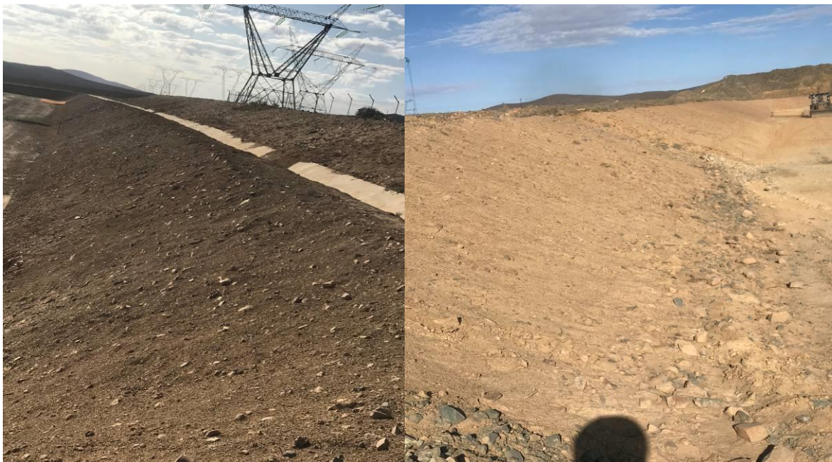
Photos: Spreading of topsoil on the 132kV and 400kV embankment.
