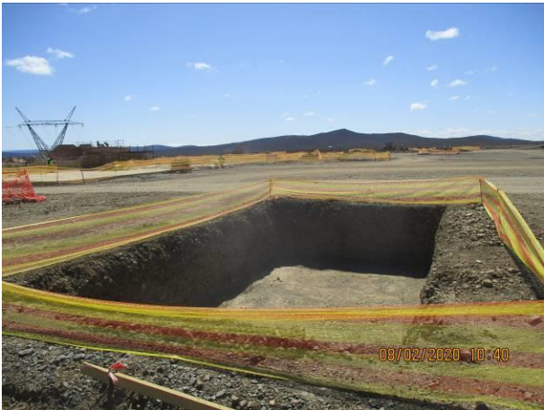
Photo: Excavated foundation.
