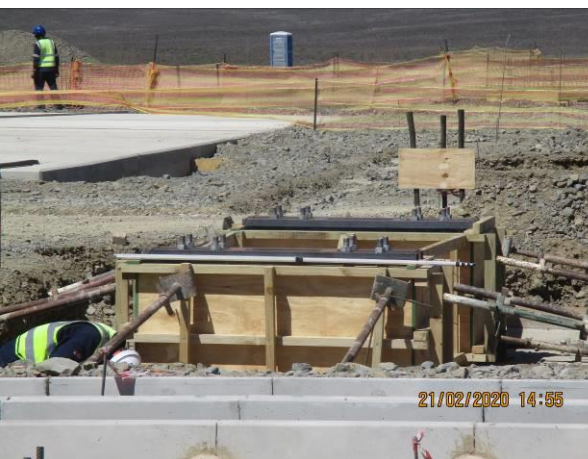
Photo: Shuttering at the foundation plinth.
