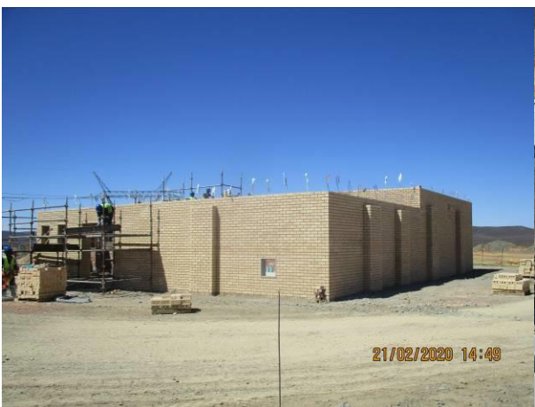
Photo: Brick work at control room building.
